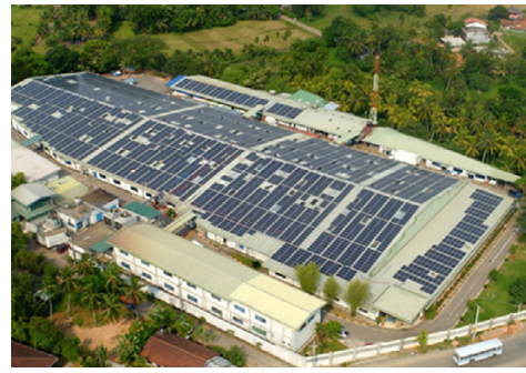
1.4MWp Solar Roof Top System, Kahathuduwa Hirdaramani Industries (Pvt) Ltd.
